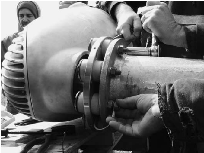
Fig. 11 Grounding turbine to tower
